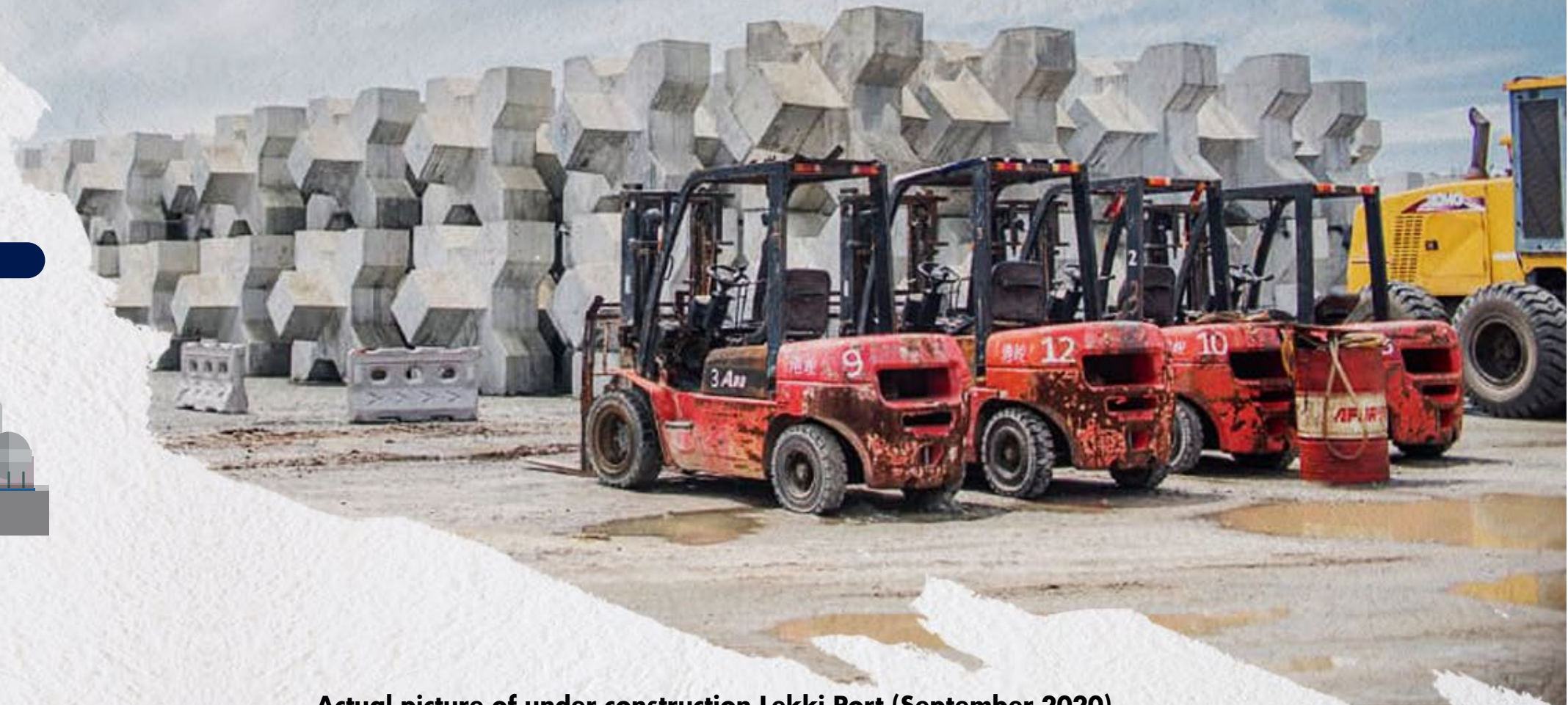
Actual picture of under construction Lekki Port (September 2020)
